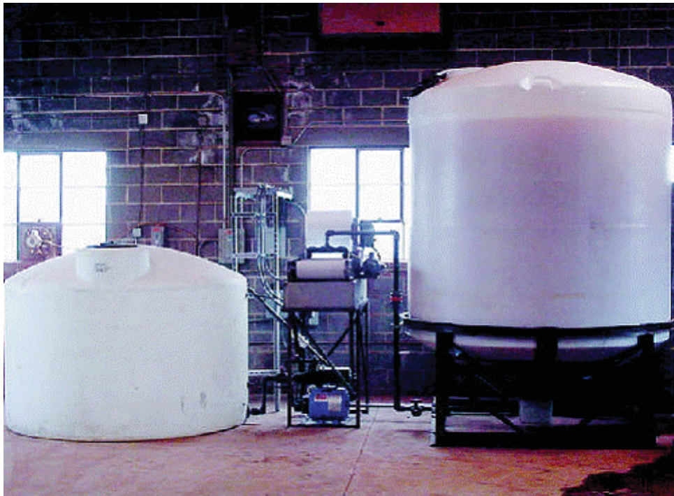
Photo. ◦ Storage tank captures used water from manufacturing process, (The Brick industry association, 2007)
